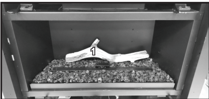
Figure 8 Log #1 Installed - COSMO36-IFT-B, DVLINEAR36, B41L-AU
