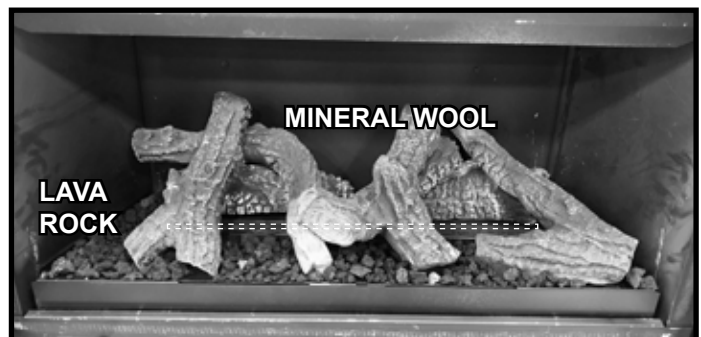
Figure 24. Properly Placed Lava Rock / Location for Mineral Wool
