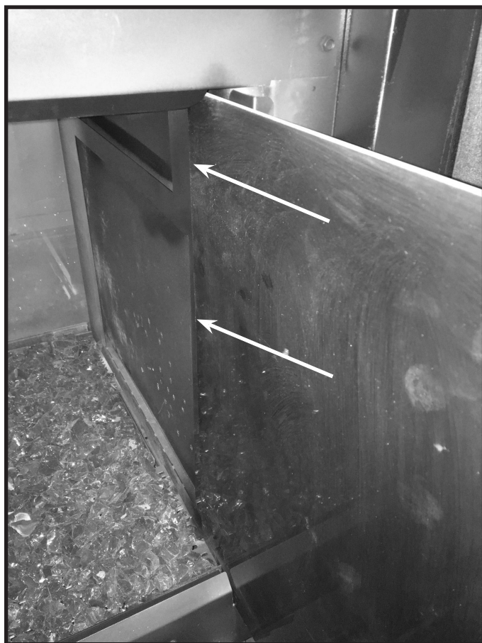
Figure 6. Rectangular Right Side Panel Installation. Shown With Optional Modern Kit Installed
