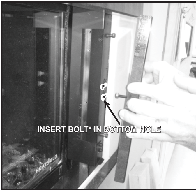
Figure 9. Install Side Granite Pieces
