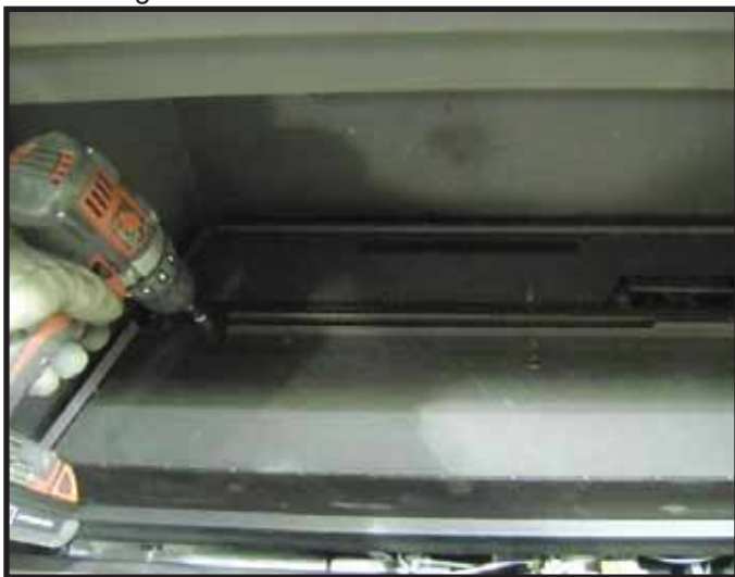
Figure 21. Install SLR-C/RAVE4013I-C Base Pan
