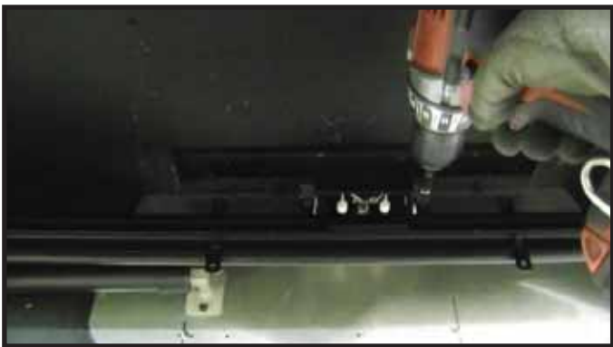
Figure 20. Install SLR-C/RAVE4013I-C Burner
