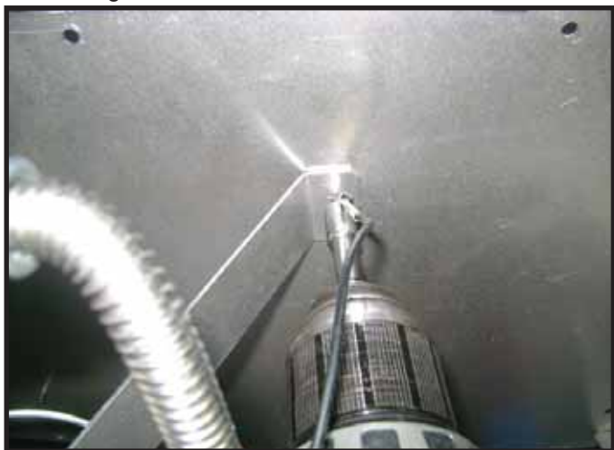
Figure 17. Attach Black Ground Wire
