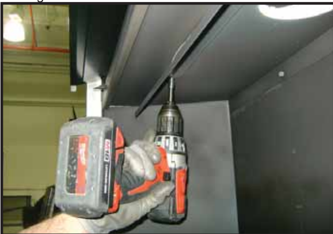
Figure 1. Remove Glass Baffle
