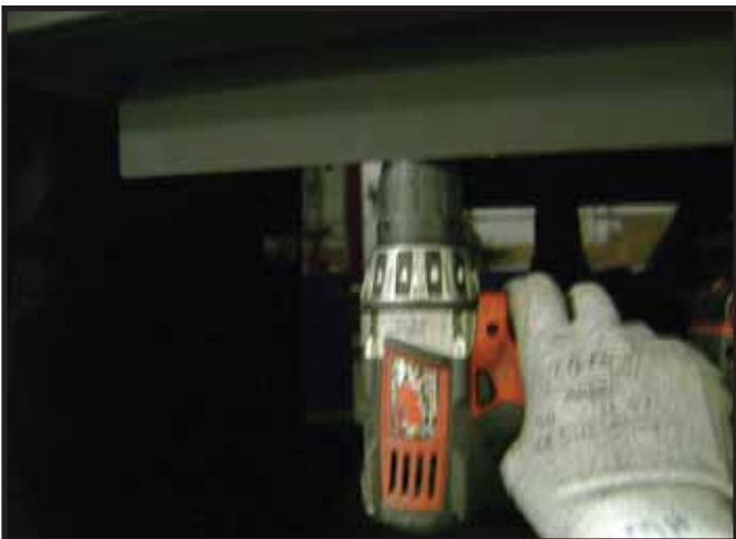
Figure 22. Install SLR-C/RAVE4013I-C Glass Baffle
