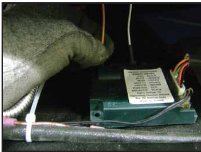
Figure 8. Disconnect Orange and White Pilot Wires
