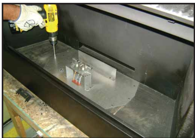
Figure 7. Remove Valve Plate
