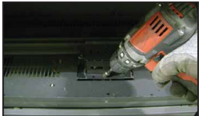
Figure 4. Remove Pilot Cover
