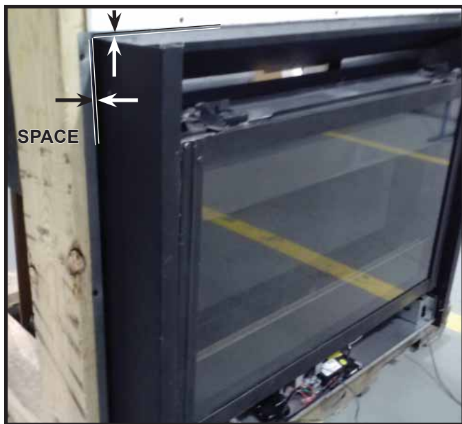
Figure 16. Splatter Guard Installation
