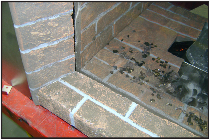
Figure 8. Outer Hearth Installation
