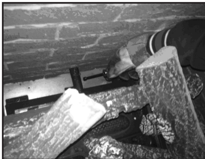
Figure 1. Air Shutter Location
