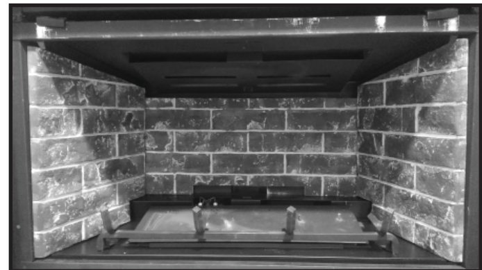
Figure 5. Refractory Panels Installed
