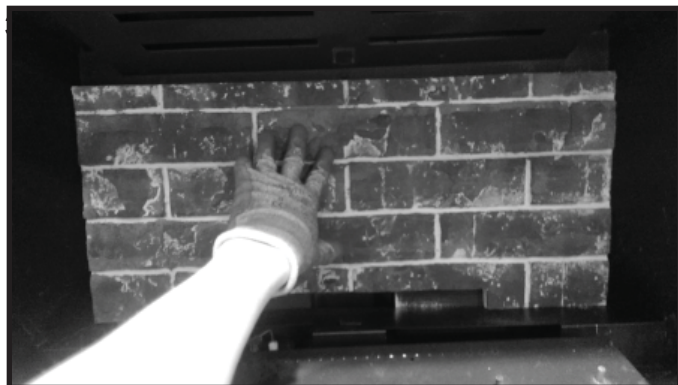
Figure 2. Install Back Refractory Panel
