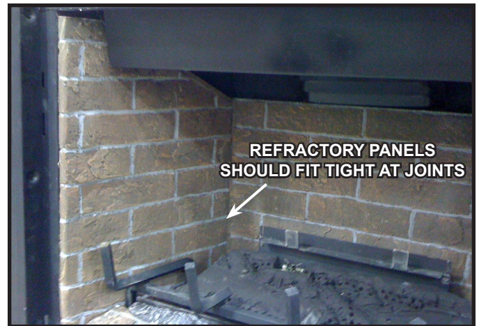
Figure 13. Side Refractory Panel Properly Installed
