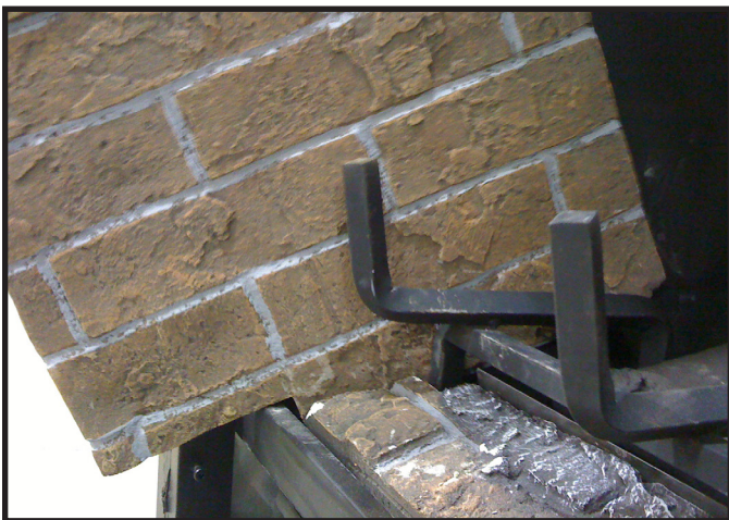
Figure 11. Left Refractory Panel Mated With Firebox Lip
