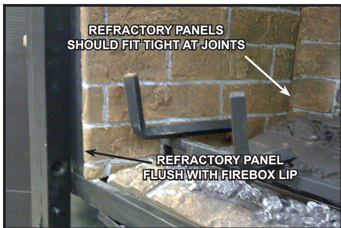
Figure 14. Check Points To Ensure Side Panel Is Properly Installed
