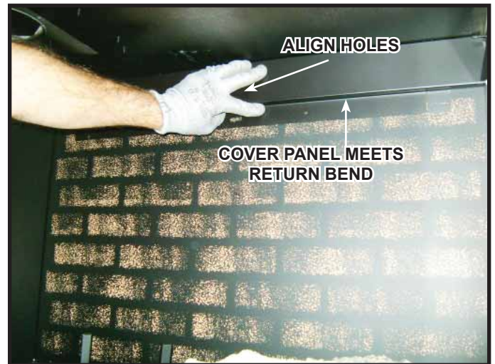
Figure 5. Install Insulation Cover Panel Top
