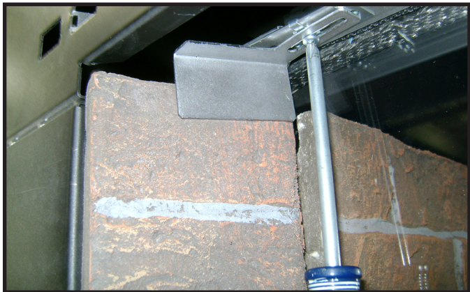
Figure 5. Installation of Refractory Brackets
