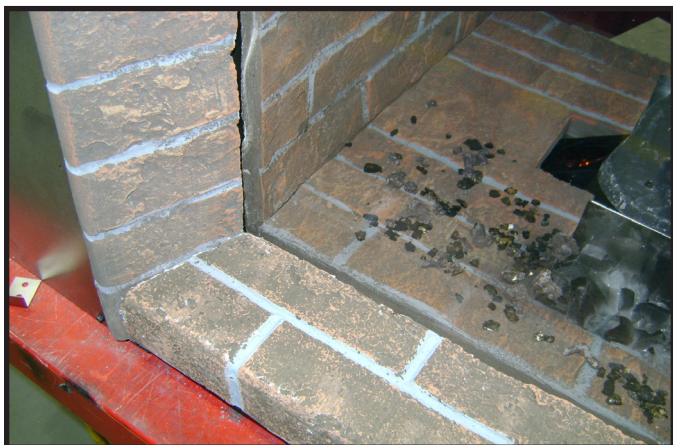
Figure 6. Installation of Outer Hearth
