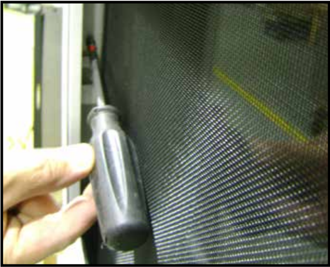
Figure 11. Tighten Phillips Screws
