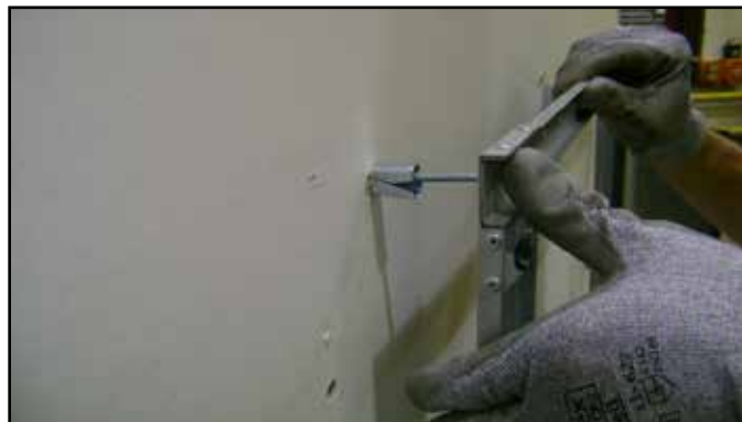
Figure 5 Installing Anchors in Hollow Wall
