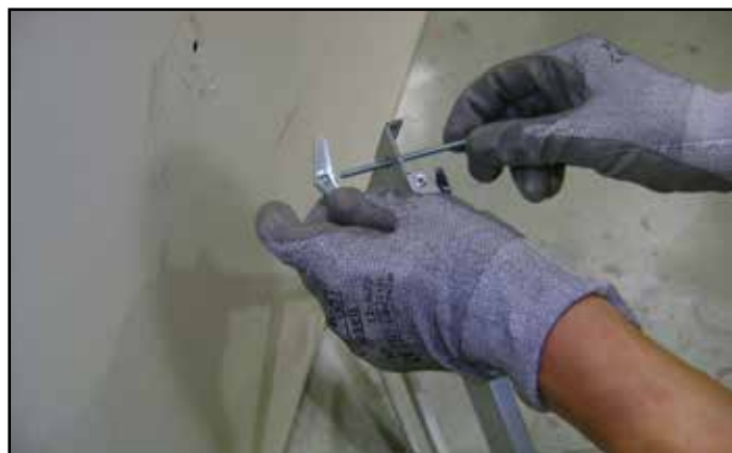
Figure 4 Toggle Bolt Installation through Mounting Bracket
