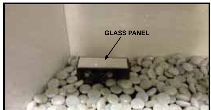
Figure 4 Install Glass Panel over Pilot Shield (Optional Glass Panel Shown)
