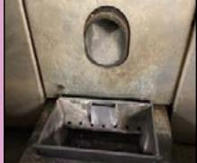
3. Remove the fire pot. Use an ash vac to remove any ash or debris in the fire pot/box area. This includes the ash over flow areas on the sides of the fire pot.
