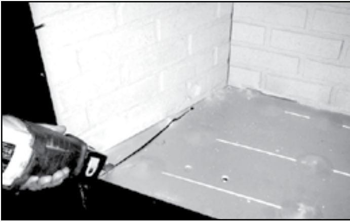
Figure 12.1 - Using a saws-all, cut out the floor.
