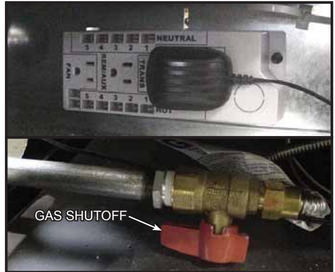
Figure 13.1 Red Gas Shutoff Knob
