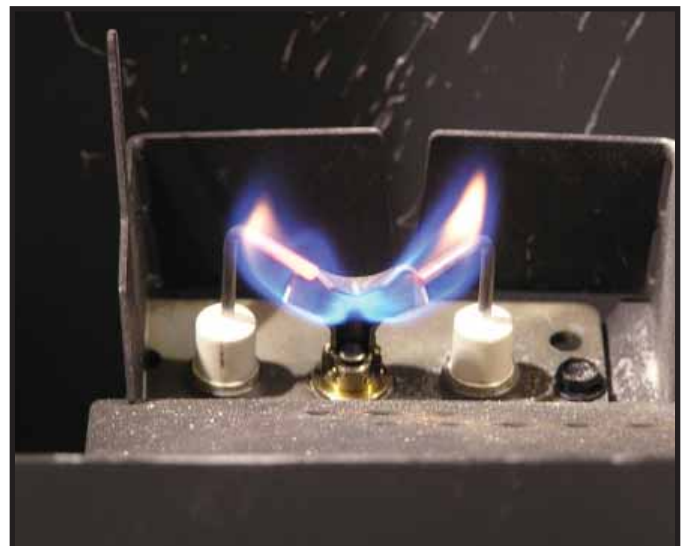
Figure 3.1 IPI Pilot Flame Pattern
