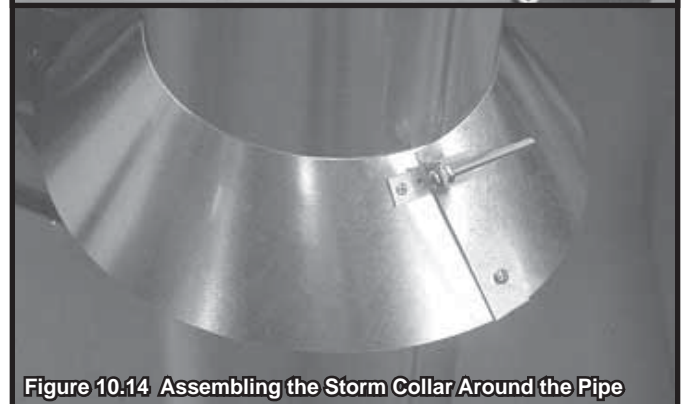
Figure 10.13 Assembling the Storm Collar
