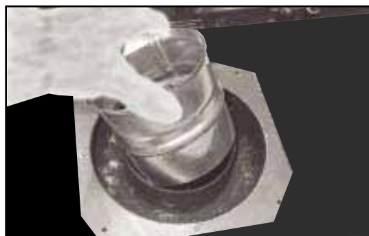
Figure 8.2 Remove the inner collar adapter.
