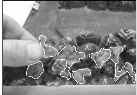
Figure 8.14 Place individual pieces of embers in front of and around the gas log where they can be seen. Space them so that gas can contact them on all sides. Avoid stacking the embers on top of each other.
