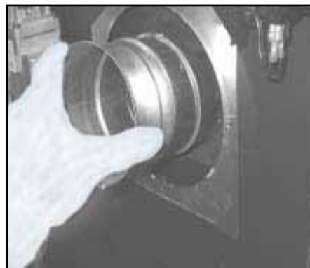
Figure 8.4 Insert the inner collar adapter to the rear vent flue.
