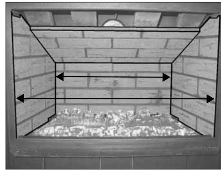
Figure 8.18 Fully installed brick set. Note that with the brick installed the firebox is narrower at the back than in the front.
