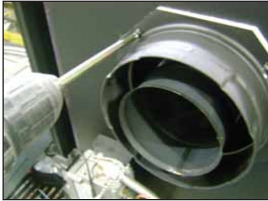
Figure 8.6 Install vent pipe adapter with gasket or high-temp silicone to rear vent opening.
