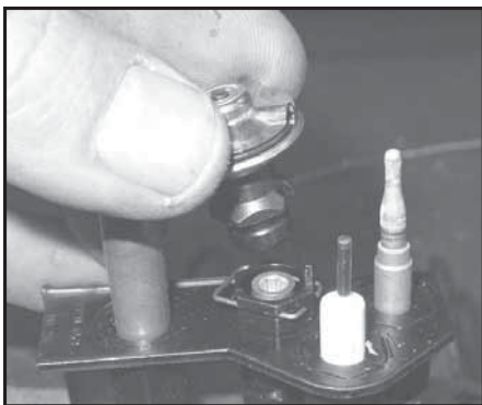
Figure 6.6 Pull off pilot hood and set it aside.
