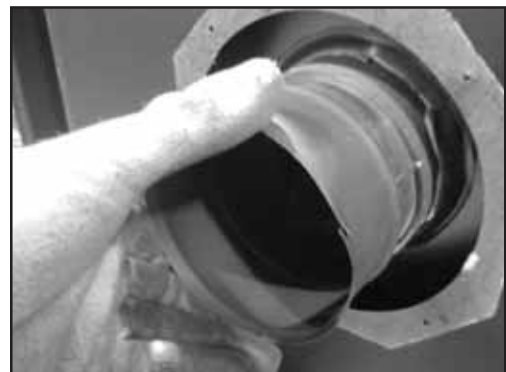
Figure 8.5 Insert inner collar adapter to rear vent flue.
