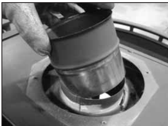
Figure 8.2 Remove inner collar adapter
