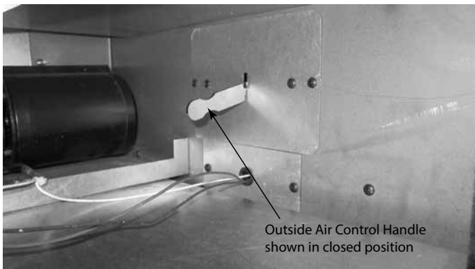
Figure 3.20 Outside Air Handle Shown on Right Side
