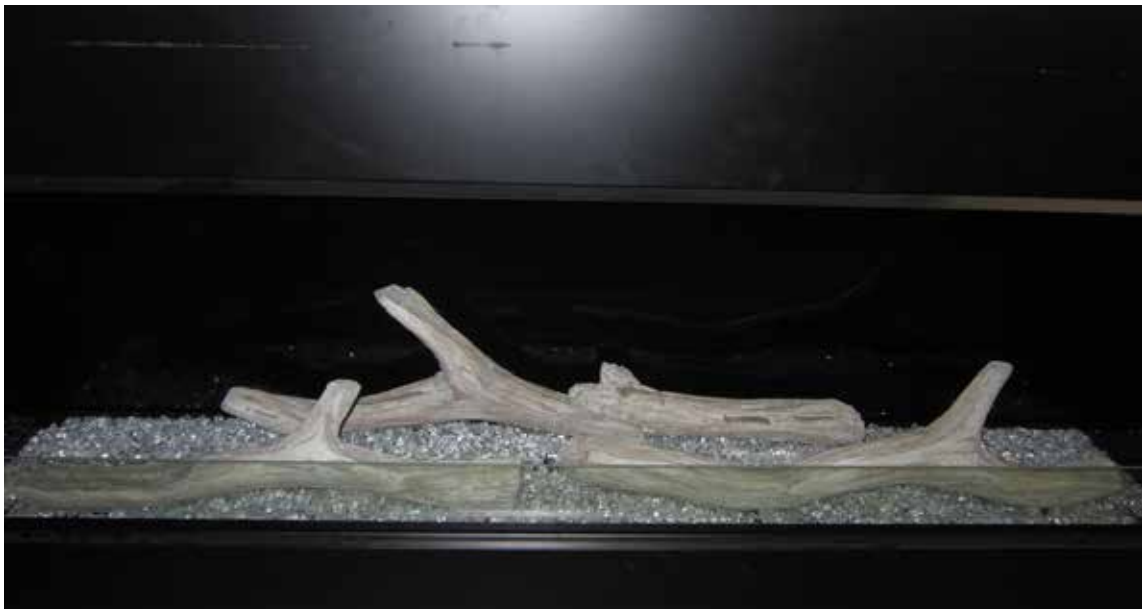
► Figure 7.8 – Log Placement for AVFL60N(P)IF AND ODLANAIG-60
