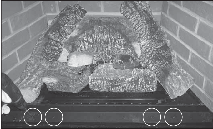
Figure 15.15 Remove Screws from Front of Hearth Pan
