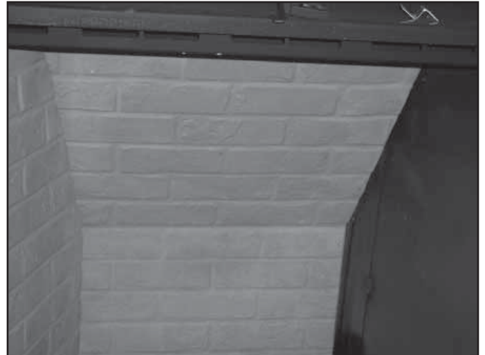
Figure 15.3 Install Upper Back Refractory
