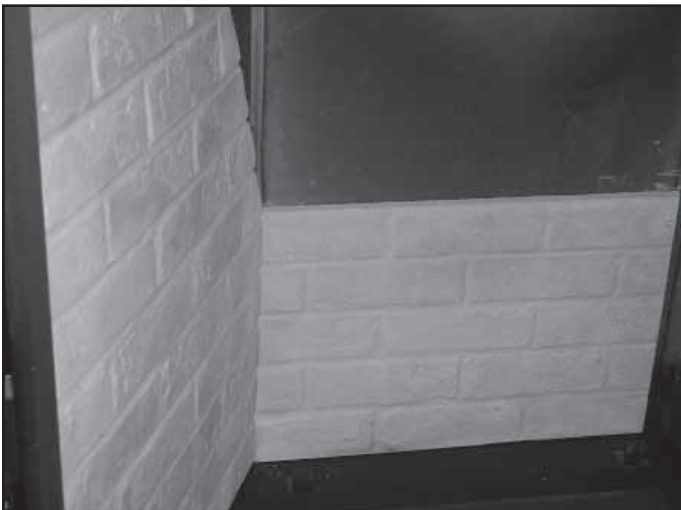
Figure 15.2 Install Lower Back Refractory
