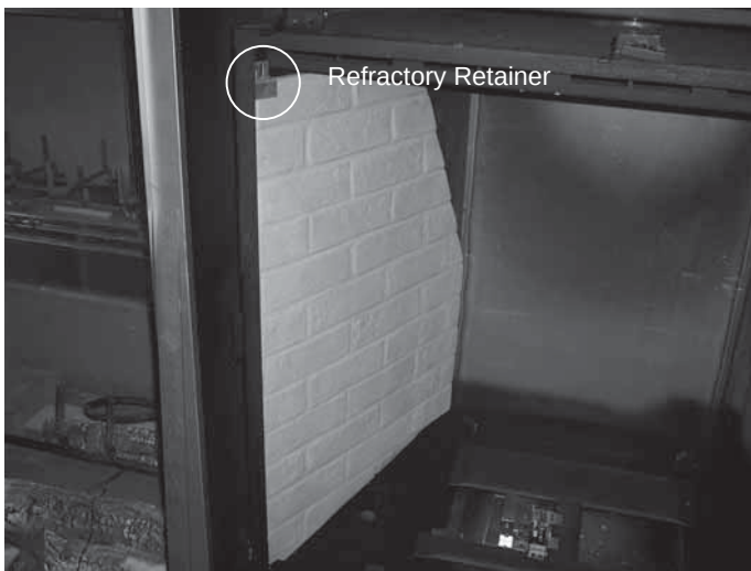
Figure 15.1 Install Left Side Refractory
