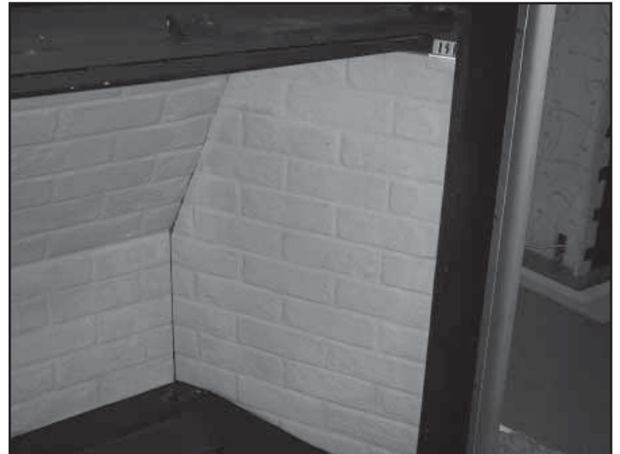
Figure 15.4 Install Right Side Refractory
