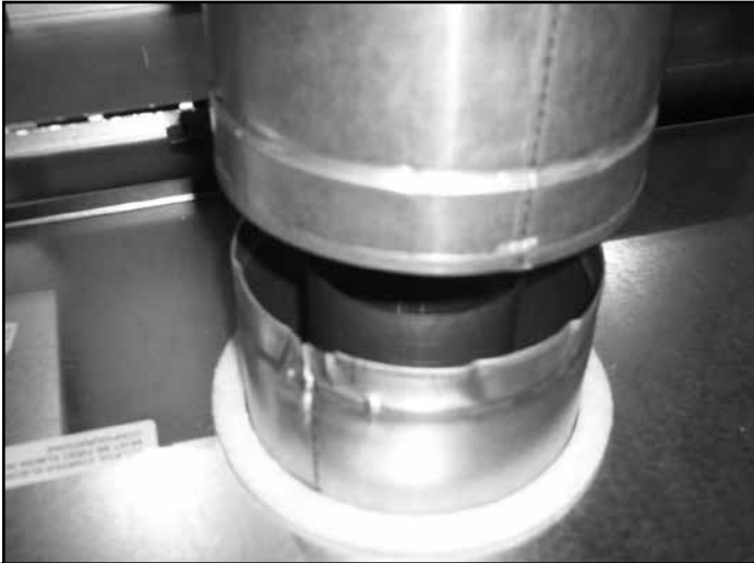
Figure 5 SLP Pipe onto SL-D Collar
