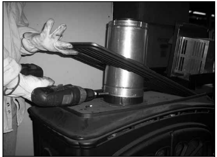
Figure 7 Fasten SLP Vent to Stove
