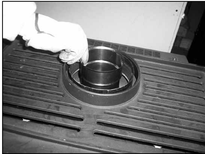
Figure 11 Install SLP-SAM Adapter
