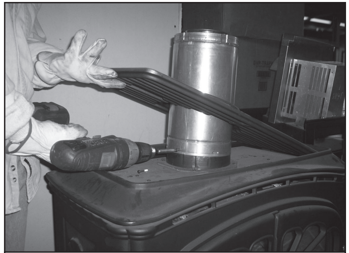
Figure 7 Fasten SLP Vent to Stove
