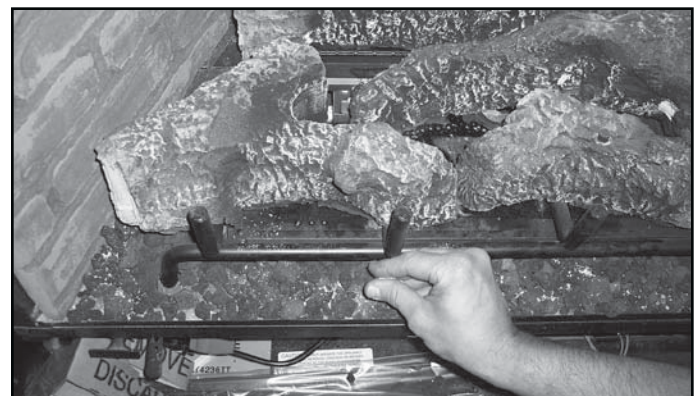
Figure 15.3 Placement of Vermiculite
