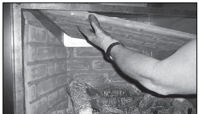
Figure 7.21 Remove Top Refractory
