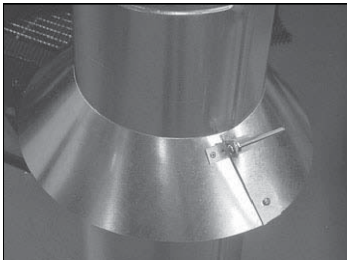
Figure 10.17 Assembling the Storm Collar Around the Pipe
