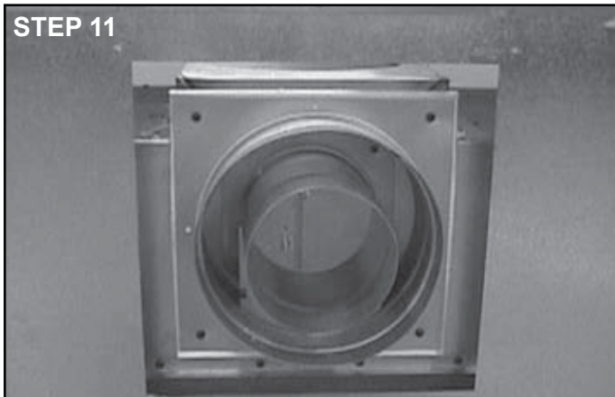
Figure 9.14 Place Outer Collar on Rear of Appliance
