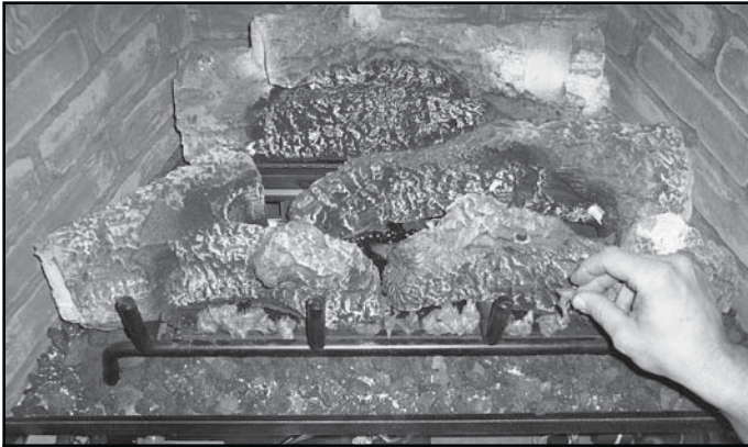
Figure 15.4 Placement of Rockwool
