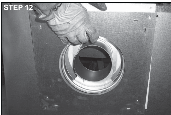
Figure 9.15 Gasket & Cover Plate Placed on Rear of Appliance
