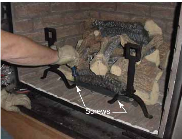
Figure 7 Position Andiron Bracket
