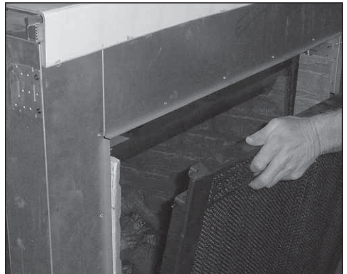
Figure 8 Installing Screen Front
