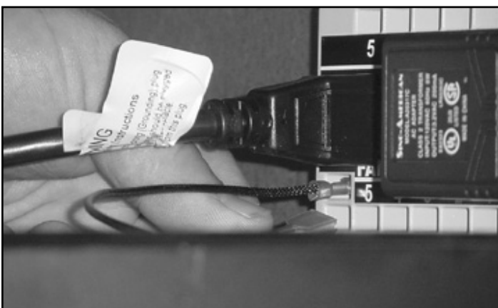
Figure 9 Jumper Wire from the Temperature Sensor Switch into Junction Box
