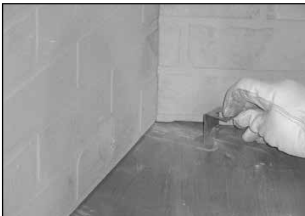
Figure 8.7 Slide Grate Retaining Bracket into Notch
