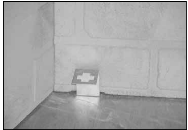
Figure 8.8 Grate Retaining Bracket in Place
