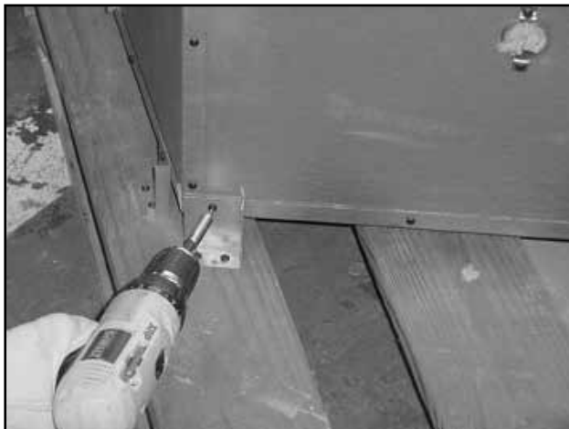
Figure 3.6 Removing Shipping Brackets
