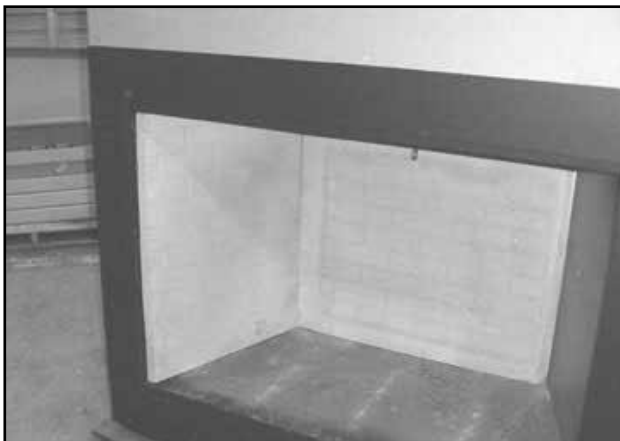
Figure 8.6 Side Refractory Installed
