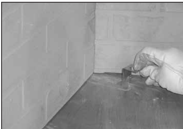
Figure 8.7 Slide Grate Retaining Bracket into Notch
