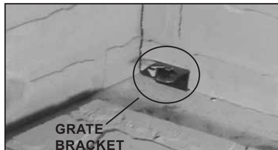
Figure 8.6 Sliding Bottom Refractory Towards Back of Fireplace
