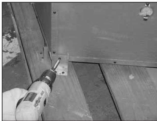
Figure 3.12 Removing Shipping Brackets
