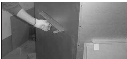
Figure 3.7 Bending Refractory Shipping Tabs Back Down
