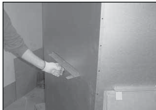
Figure 7.2 Bending Refractory Shipping Tabs Back Down
