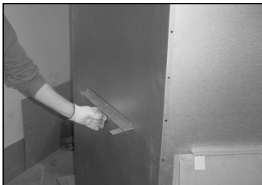
Figure 4.6 Bending Refractory Shipping Tabs Back Down
