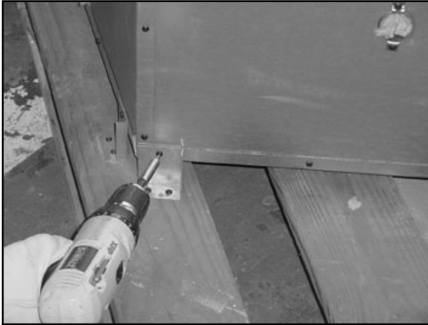
Figure 4.11 Removing Shipping Brackets
