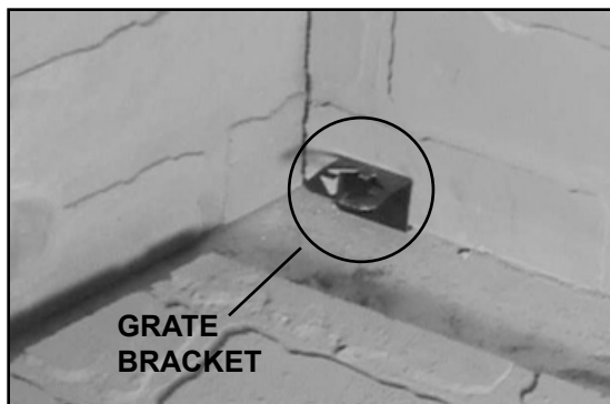
Figure 4.16 Sliding Bottom Refractory Towards Back of Fireplace
