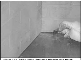
Figure 7.15 Slide Grate Retaining Bracket into Notch
