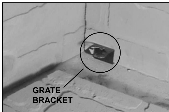
Figure 4.16 Sliding Bottom Refractory Towards Back of Fireplace
