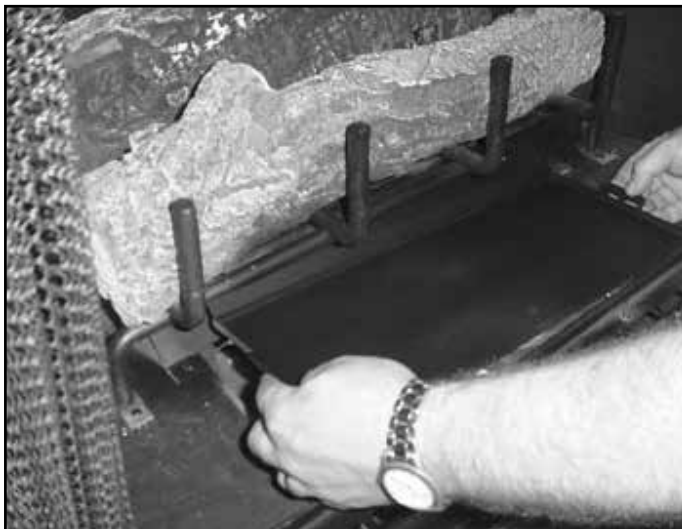
Figure 14.2 Control Access Panel Installation/Removal
