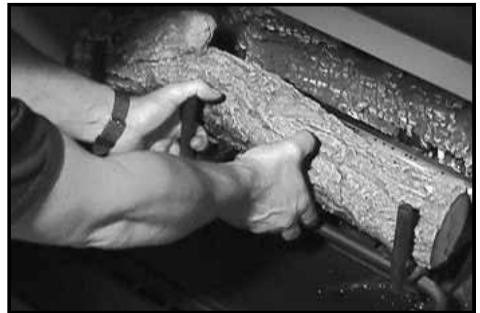
Figure 14.7 Remove Grate/Log Assy.
