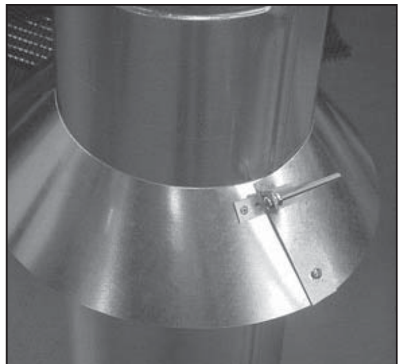
Figure 8.17 Assembling the Storm Collar Around the Pipe
