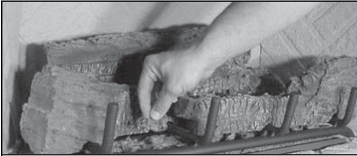
Figure 12.3 Placing the Rockwool
