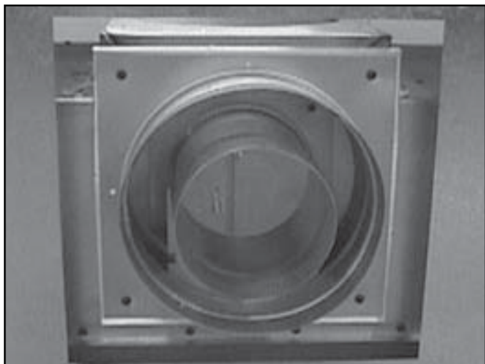
Figure 7.10 Remove Inner Cover Plate
