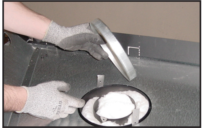
Figure 7.4 Remove the seal cap.
