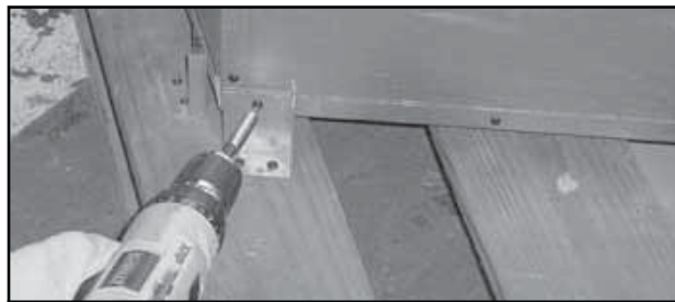
Figure 7.6 Removing Shipping Brackets
