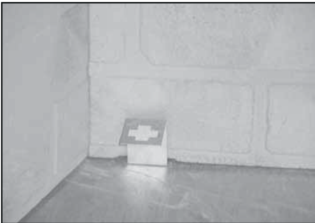
Figure 7.16 Grate Retaining Bracket in Place
