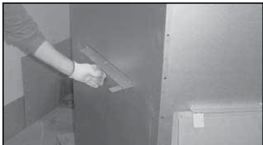
Figure 7.2 Bend Refractory Brackets Back Down
