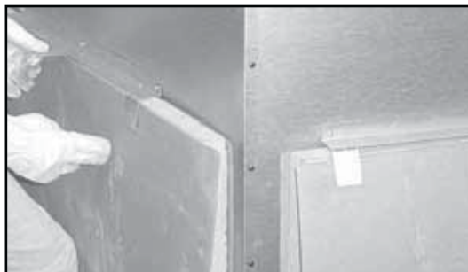
Figure 7.1 Unpack Back Refractory
