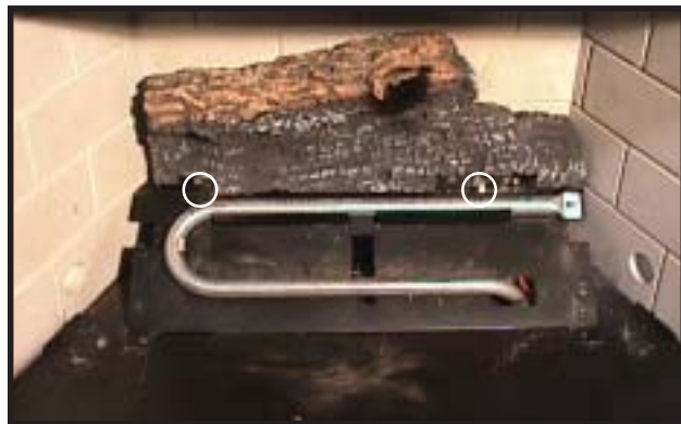
Figure 28 Back Log Removal
