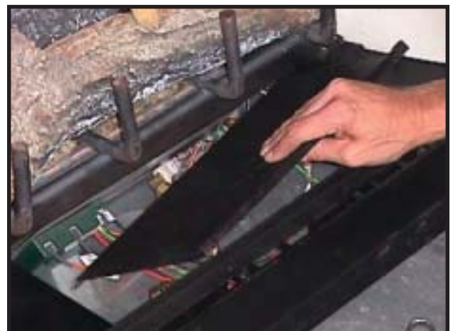
Figure 16 - Control Access Panel Installation/ Removal
