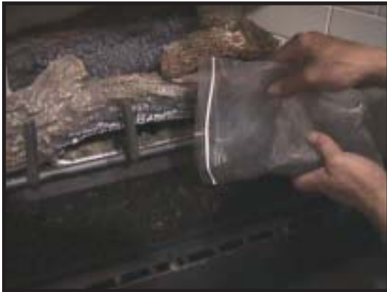
Figure 17 Placing the Lava Rock
