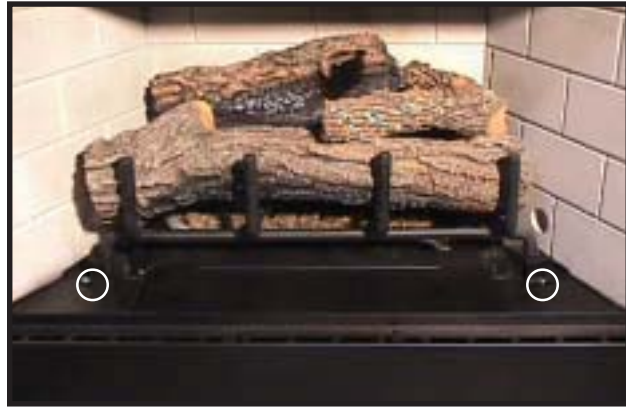
Figure 26 Unscrewing the Log/Grate Assembly from the Hearth Pan
