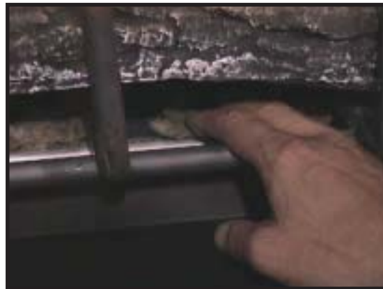
Figure 19 Placing the Rock Wool
