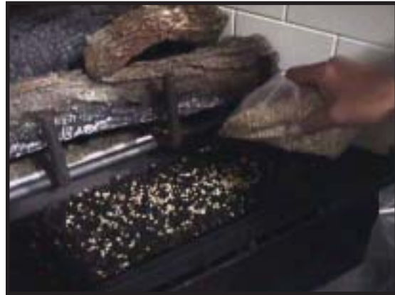
Figure 18 Placing the Vermiculite
