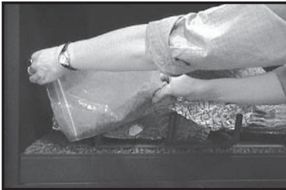
Figure 60 - Placing the Lava Rock
