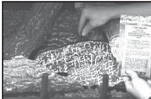
Figure 63 - Placing the Fire Glow
