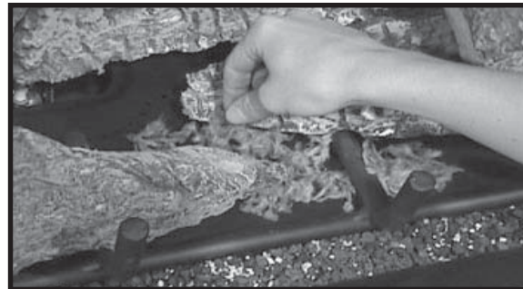
Figure 62 - Placing the Rock Wool
