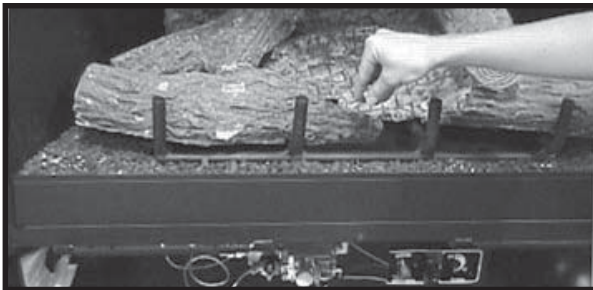
Figure 61 - Placing the Vermiculite
