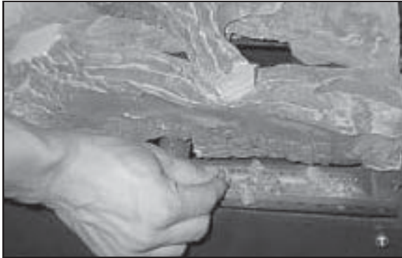
Figure 23 - Placing the Rock Wool
