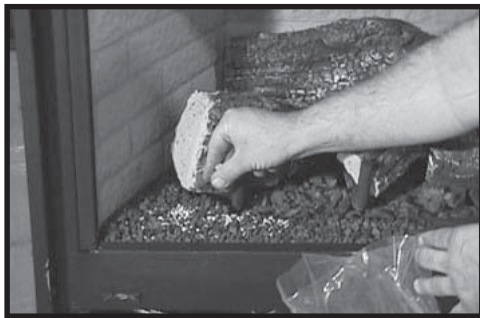
Figure 45 - Placing the Vermiculite
