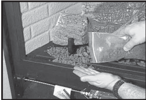
Figure 44 - Placing the Lava Rock
