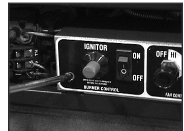
Figure 3BF Replacing Switch onto Bracket
