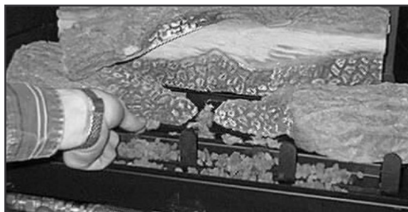
Figure 16 - Placing Rock Wool
