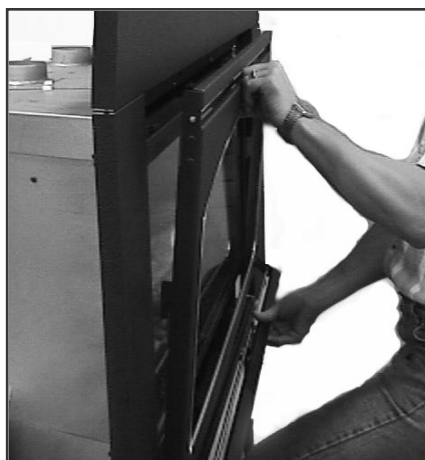
Figure 1AF - Placing Front Face into Slots
