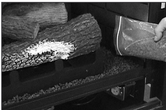
Figure 15 - Placing Lava Rock
