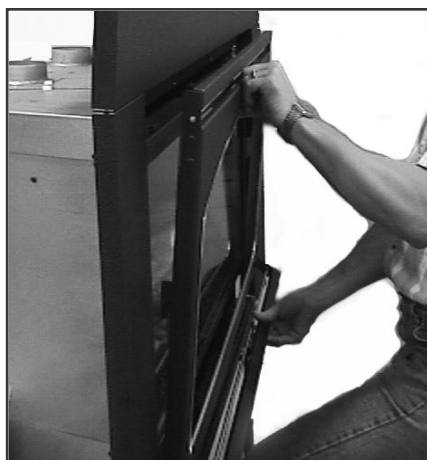
Figure 1AF - Placing Front Face into Slots
