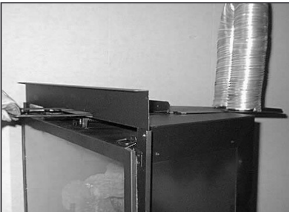
Figure 4 - Reinstalling the Starter Collar
