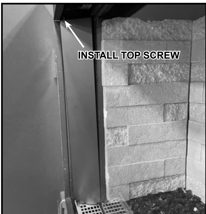
Figure 4.11 Transition Panel installed
