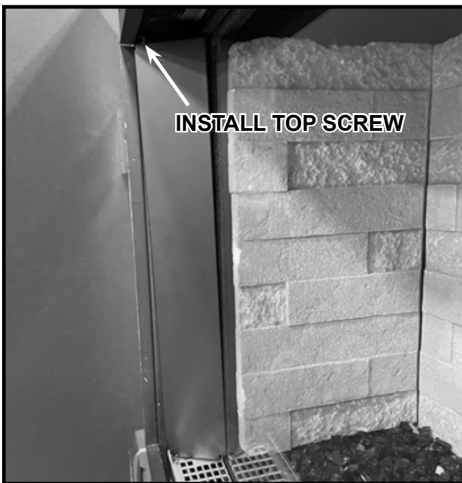
Figure 11.21 Transition Panel installed
