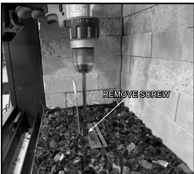
Figure 11.4 Place Media, Remove Media Placement Jig Screw
