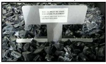
Figure 9.9 Rock Placement Jig
