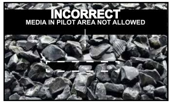
Figure 9.11 INCORRECT Media Placement
