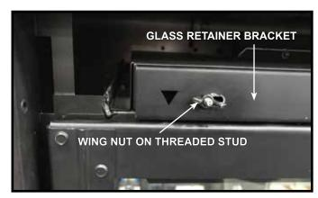
9.3 Glass Retainer Bracket & Wing Nut Detail
