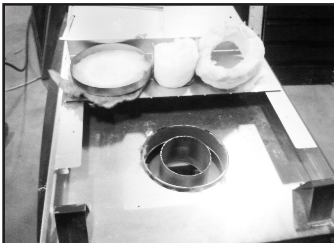
Figure 6.5 Remove and discard the seal cap, insulation donut, insulation plug, and the insulation basket. Attach the first vent section (it will snap into place). Slide the vent gasket onto the vent section and then, up against the appliance. Secure the vent gasket to the appliance with two self-tapping screws found in the manual bag. Note: The vent gasket can found in the manual bag.
